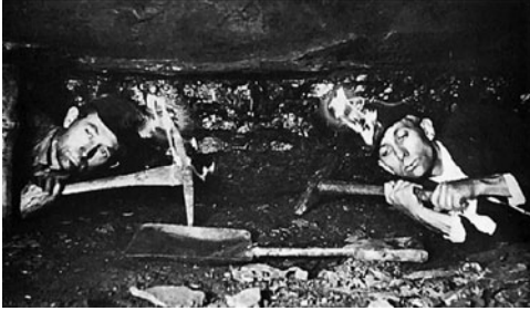
Fig. 16.7.2 Workers in underground coal mine.
