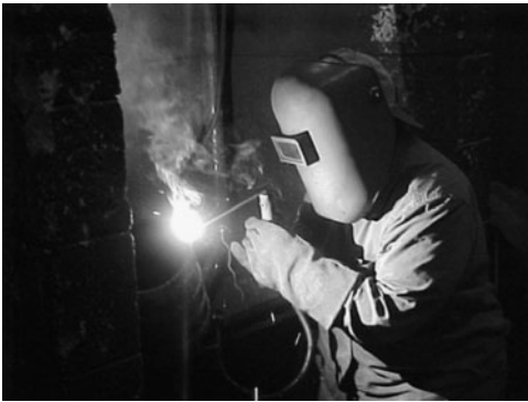
Fig. 16.7.3 A welder at work.
