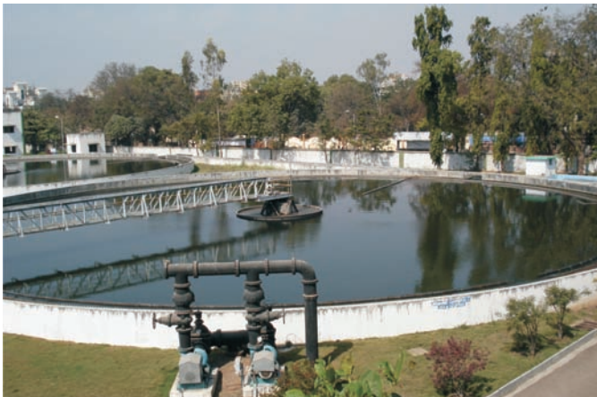
Primary Sedimentation Tank
