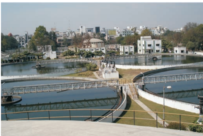
Secondary Sedimentation Tank
